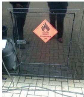
This shows warning signage on a locked gas compartment but no evidence of ventilation.
