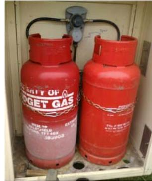
Frosting on the bottle caused by excessive cooling effect due to gas being drawn off too quickly.
