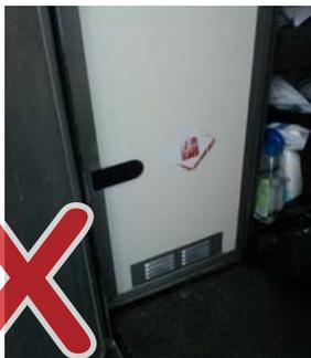
This shows a gas compartment venting and opening into the cooking area in a unit.
