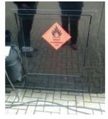
This shows warning signage on a locked gas compartment but no evidence of ventilation.
