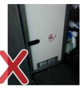
This shows a gas compartment venting and opening into the cooking area in a unit.
