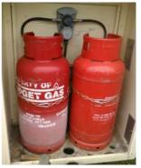
Frosting on the bottle caused by excessive cooling effect due to gas being drawn off too quickly.
